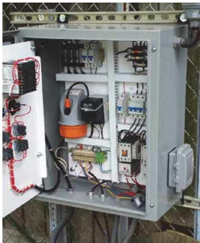
A standard SCADA installation for the Harris County Water Control and Improvement District No. 1 includes a remote telemetry unit (RTU) – the grey cylinder with the orange base – installed in a control cabinet. The RTU takes up very little space and uses cellular technology to communicate with the cloud-based system. Harris County Water Control and Improvement District No. 1
